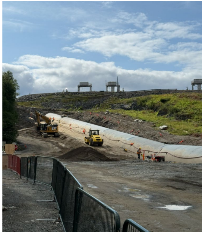
Figure 7: Placing Common Backfill on South Side of Penstock
