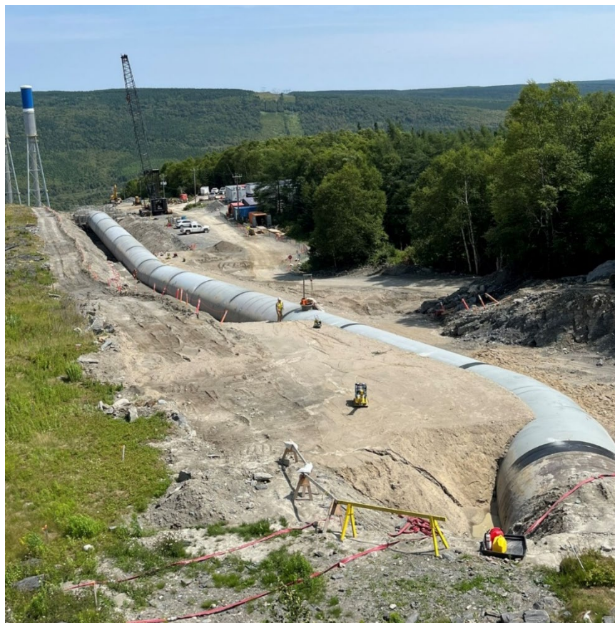
Figure 8: Placing Common Backfill on North Side of Penstock
