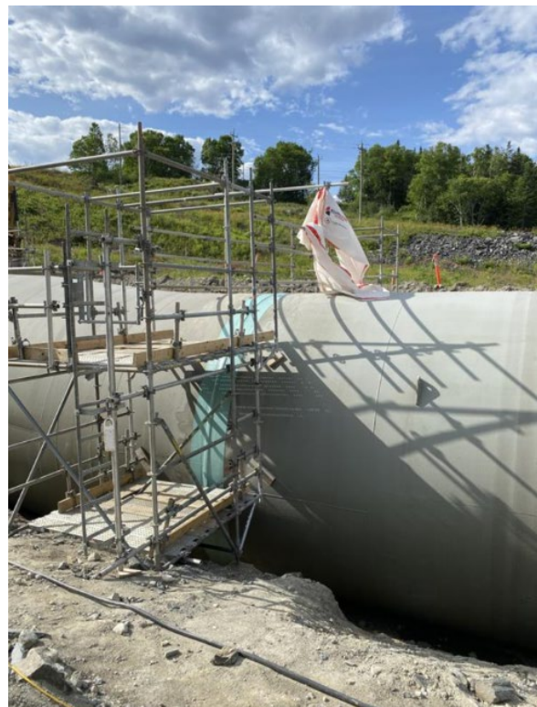
Figure 5: Installation of Exterior Coating Wrap on Cans 8 and 9
