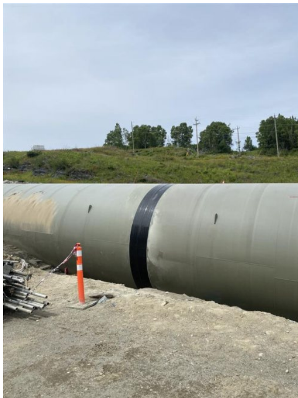
Figure 5: Installation of Exterior Coating Wrap on Cans 8 and 9
